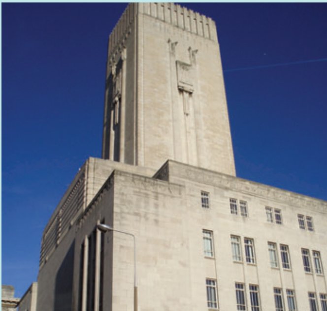
Georges Dock tunnel ventilation and control station
